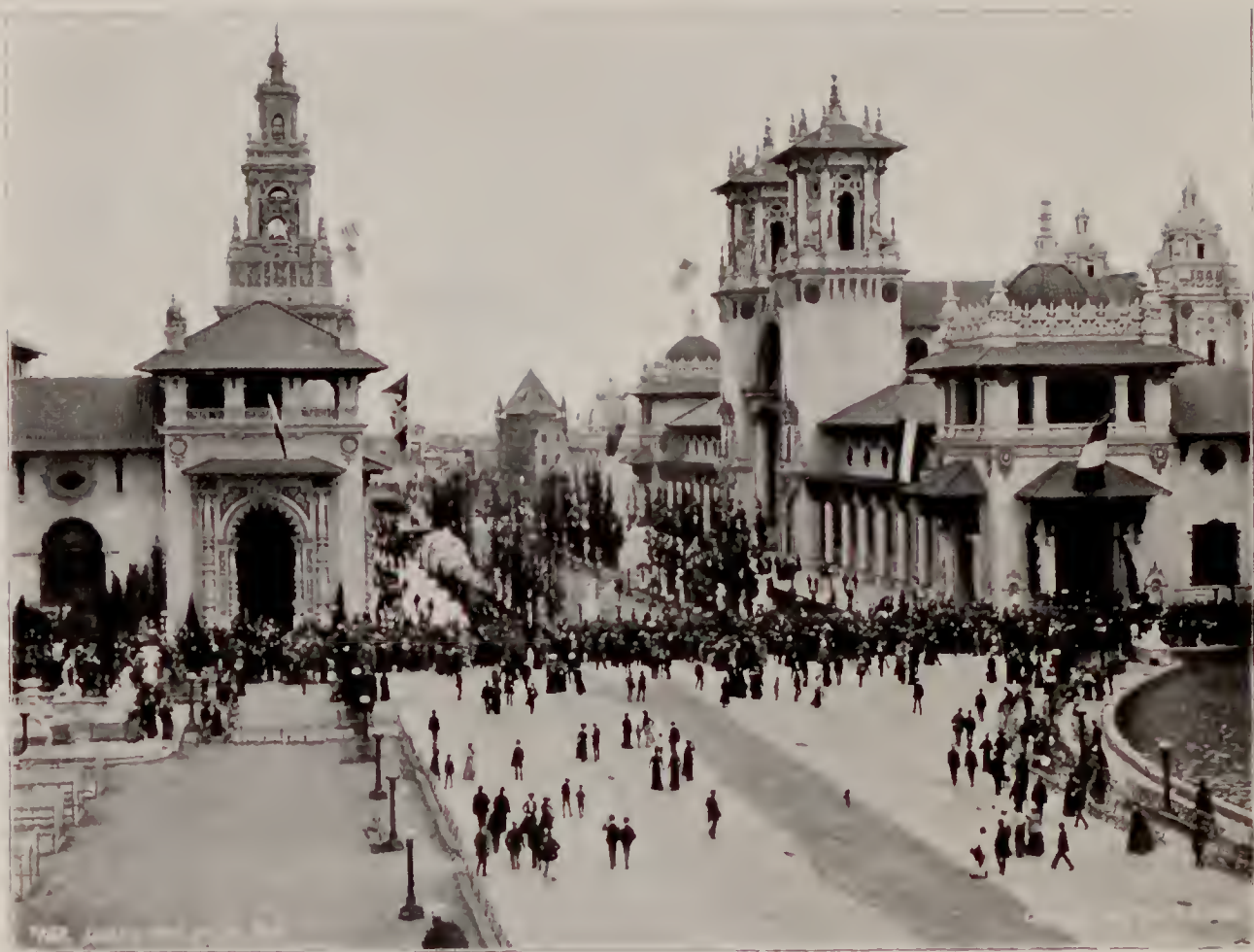
LOOKING WEST ON THE MALL.—On the right is the Electricity Building, on the left Machinery. Between them is a beautiful Sunken Garden adorned with statuary, rows of poplar trees, shrubs and flowering plants. In the distance is Alt Nürnberg on the Midway.
